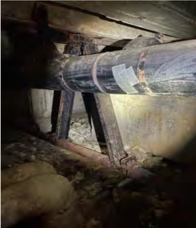
Cloth wrapped black pipe in crawlspace
