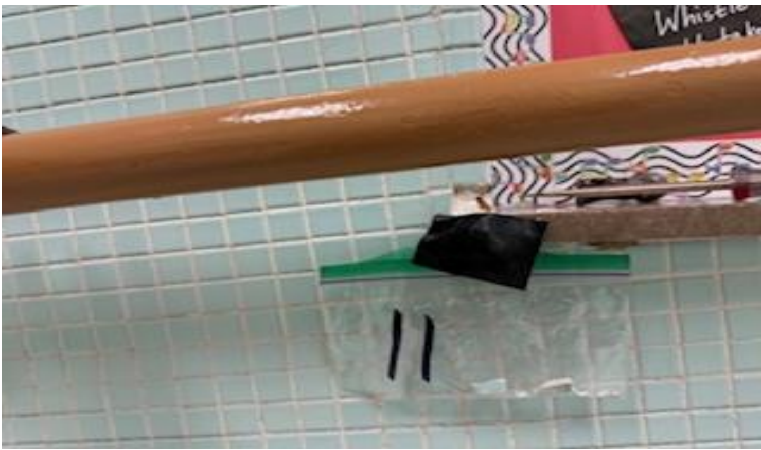
9. VIEW OF REPRESENTATIVE (TYPICAL) SAMPLE OF NON-ACM GREENISH WALL CERAMIC TILES AND GROUT LOCATED ON VARIOUS INTERIOR WALL SURFACES THROUGHOUT THE BUILDINGS AT THOMAS C. MARSH PREPARATORY ACADEMY
