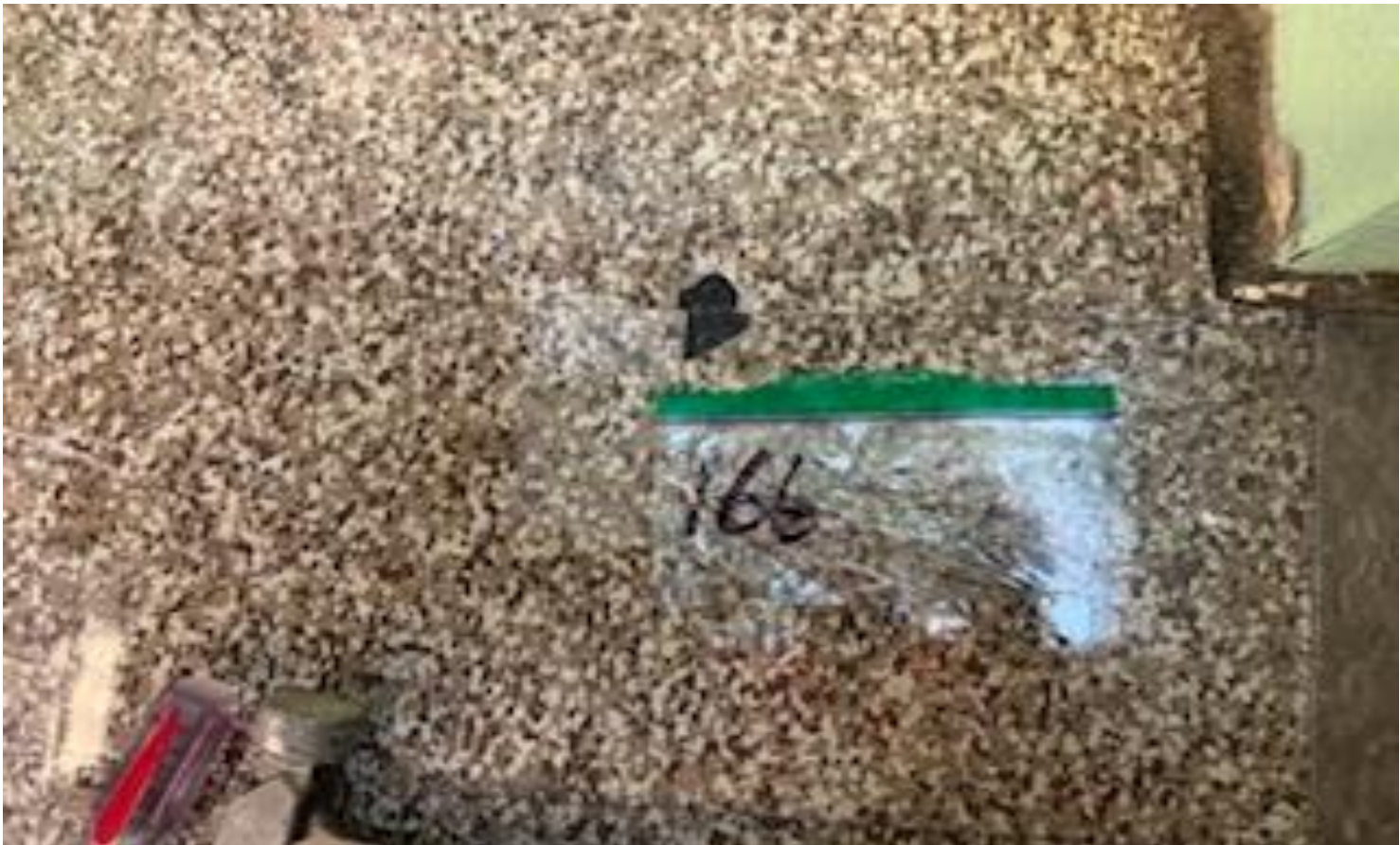
68. VIEW OF MORE REPRESENTATIVE (TYPICAL) SAMPLE OF ACM DARK BROWN 9" X 9" FLOOR TILES AND BLACK MASTIC LOCATED CLASS ROOMS ON THE 3 RD FLOOR SURFACES IN BUILDINGS AT THOMAS C. MARSH PREPARATORY ACADEMY
