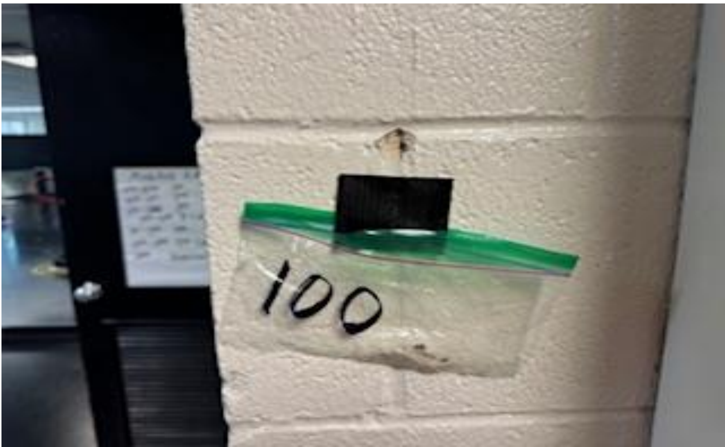
51 VIEW OF MORE REPRESENTATIVE (TYPICAL) SAMPLE OF NON-ACM CONCRETE MASONRY UNITS (CMU) AND MORTAR LOCATED THROUGHOUT INTERIOR WALL SURFACES IN BUILDINGS AT THOMAS C. MARSH PREPARATORY ACADEMY
