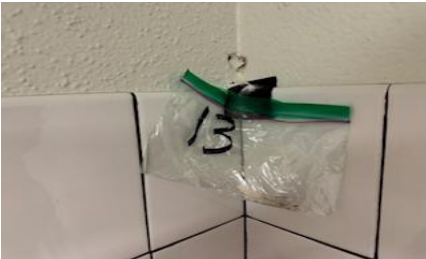
10. VIEW OF REPRESENTATIVE (TYPICAL) SAMPLE OF NON-ACM PLASTER WALL LOCATED THROUGHOUT INTERIOR WALL SURFACES IN BUILDINGS AT THOMAS C. MARSH PREPARATORY ACADEMY
