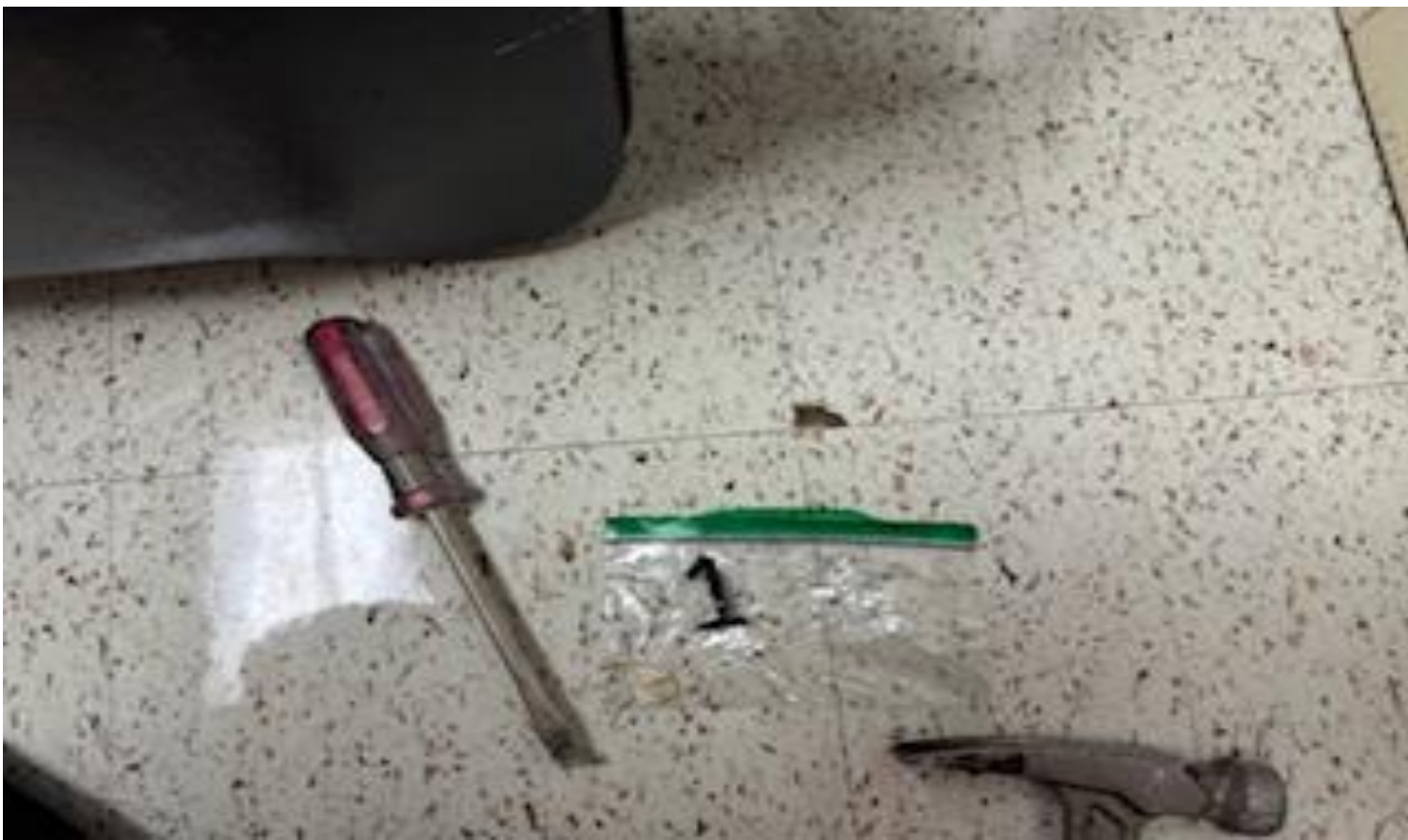
1. VIEW OF REPRESENTATIVE (TYPICAL) SAMPLE OF NON-ACM 12" X12" FLOOR TILES AND MASTIC LOCATED THROUGHOUT INTERIOR FLOOR SPACES IN BUILDINGS AT THOMAS C. MARSH PREPARATORY ACADEMY
