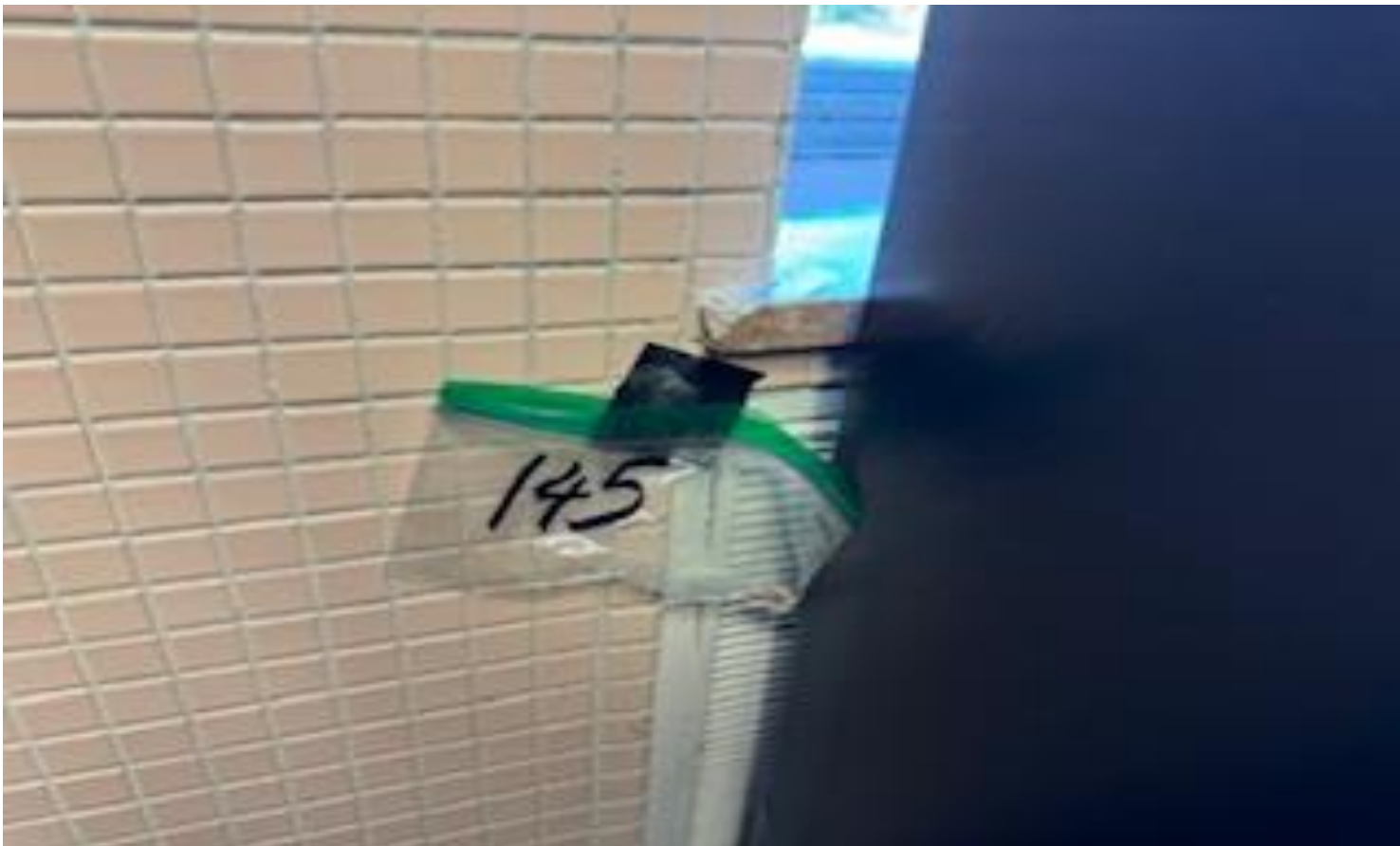
62. VIEW OF REPRESENTATIVE (TYPICAL) SAMPLE OF NON-ACM WINDOW SILL CERAMIC TILES AND GROUT LOCATED THROUGHOUT THE BUILDINGS AT THOMAS C. MARSH PREPARATORY ACADEMY
