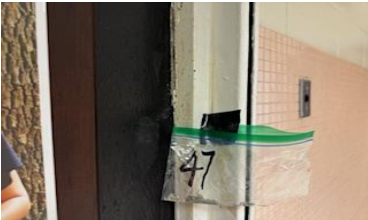
33. VIEW OF MORE REPRESENTATIVE (TYPICAL) SAMPLE OF NON-ACM BUILDING DEMARCATION SEALANT LOCATED ON VARIOUS INTERIOR WALL SURFACES THROUGHOUT THE BUILDINGS AT THOMAS C. MARSH PREPARATORY ACADEMY
