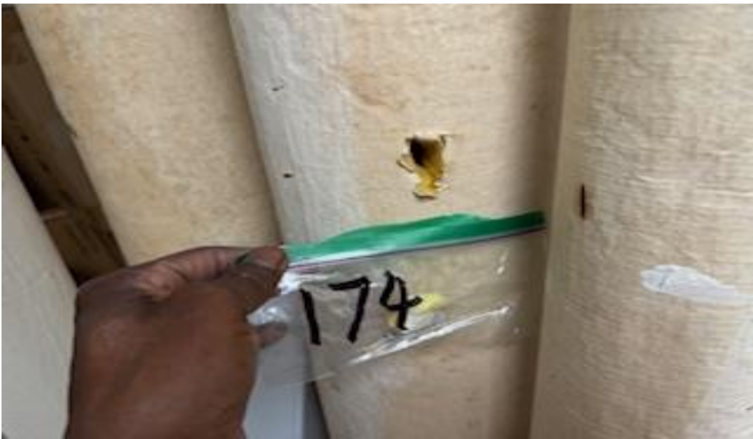
69 VIEW OF REPRESENTATIVE (TYPICAL) PHOTOGRAPHS OF NON-ACM TSI WHITE WRAP AND WHITE MASTIC LOCATED IN STORAGE ROOMS ON THE 3 RD FLOOR IN BUILDINGS AT THE THOMAS C. MARSH PREPARATORY ACADEMY
