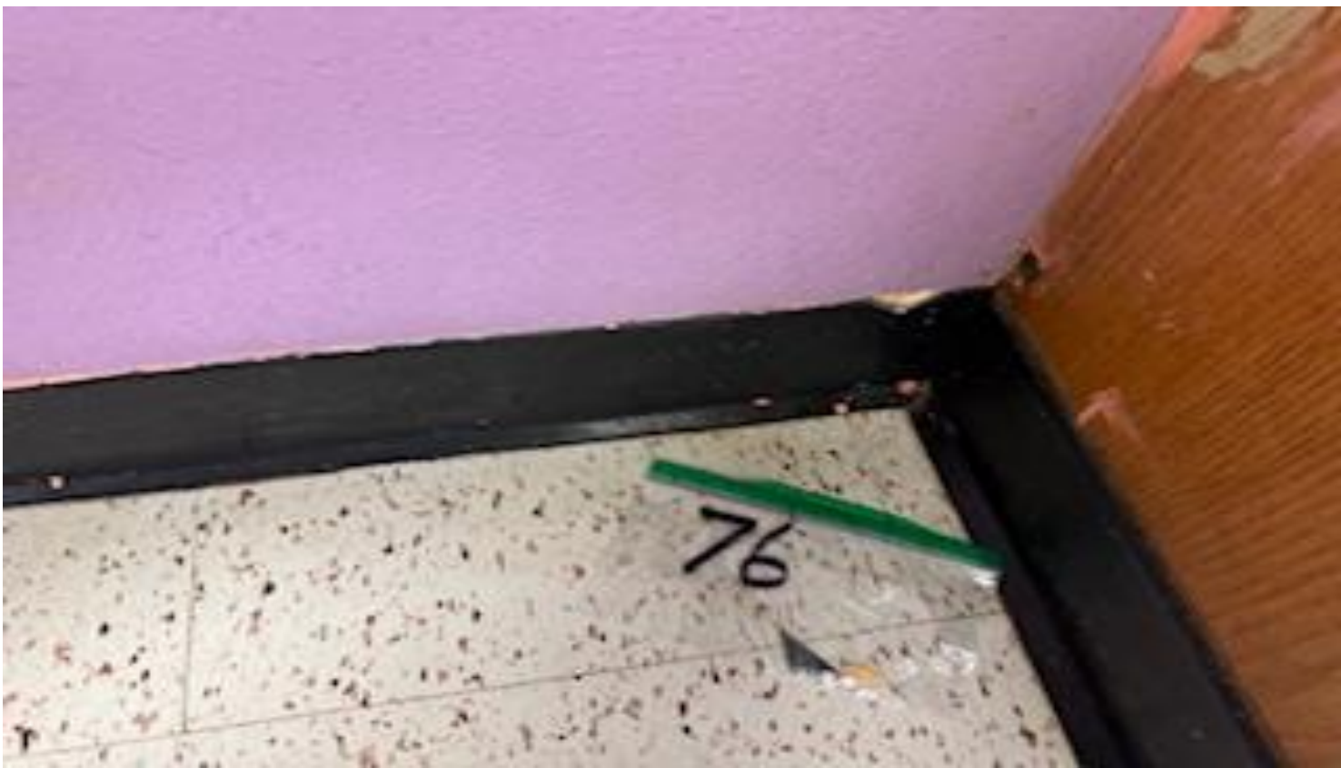
45. VIEW OF REPRESENTATIVE (TYPICAL) SAMPLE OF NON-ACM MASTIC UNDERNEATH RUBBER COVE-BASE LOCATED ON INTERIOR BOTTOM WALLS THROUGHOUT THE BUILDING AT THOMAS C. MARSH PREPARATORY ACADEMY
