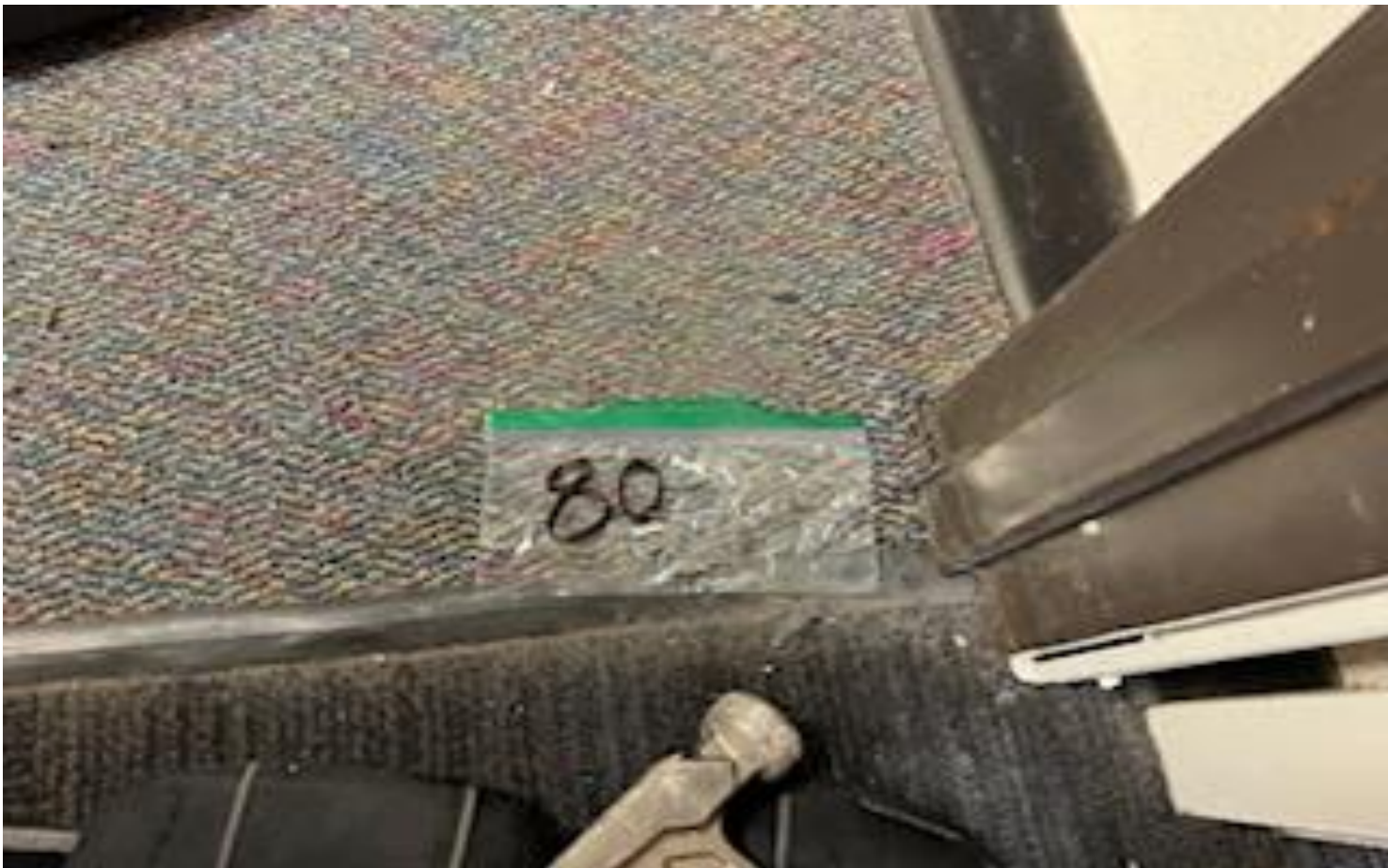
46. VIEW OF REPRESENTATIVE (TYPICAL) SAMPLE OF NON-ACM CARPET GLUE LOCATED IN VARIOUS EXECUTIVE OFFICE AND ELSEWHERE IN BUILDINGS AT THOMAS C. MARSH PREPARATORY ACADEMY
