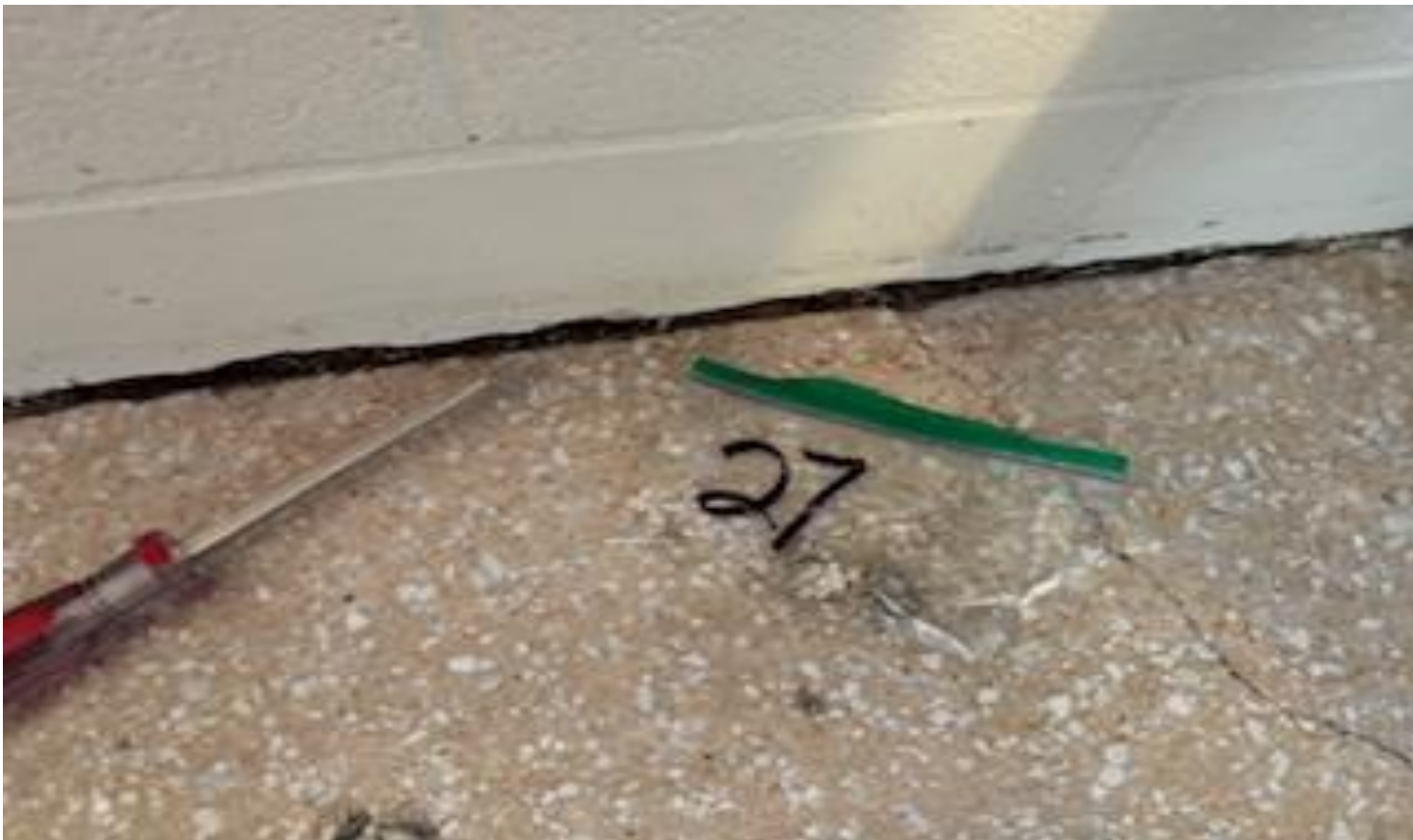
20. VIEW OF REPRESENTATION (TYPICAL) SAMPLE OF NON-ACM TERRAZZO FLOORING LOCATED IN VARIOUS WET SURFACES THROUGHOUT THE BUILDINGS AT THOMAS C. MARSH PREPARATORY ACADEMY
