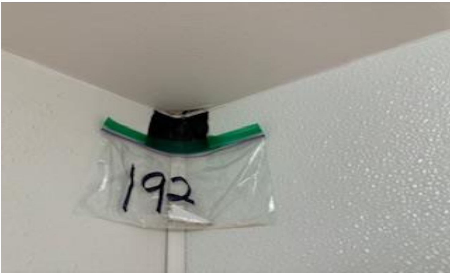
75. VIEW OF REPRESENTATIVE (TYPICAL) SAMPLE OF NON-ACM CEILING TEXTURE JOINT COMPOUND AND SHEETROCK MUD LOCATED ON CEILING SURFACES ON THE 3 RD FLOOR IN BUILDINGS AT THOMAS C. MARSH PREPARATORY ACADEMY
