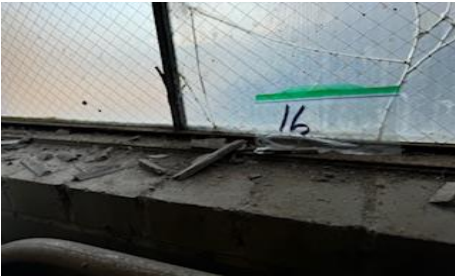
12. VIEW OF REPRESENTATIVE (TYPICAL) SAMPLE OF ACM WINDOW GLASS PANES GLAZING LOCATED THROUGHOUT INTERIOR WINDOW SURFACES IN BUILDINGS AT THOMAS C. MARSH PREPARATORY ACADEMY
