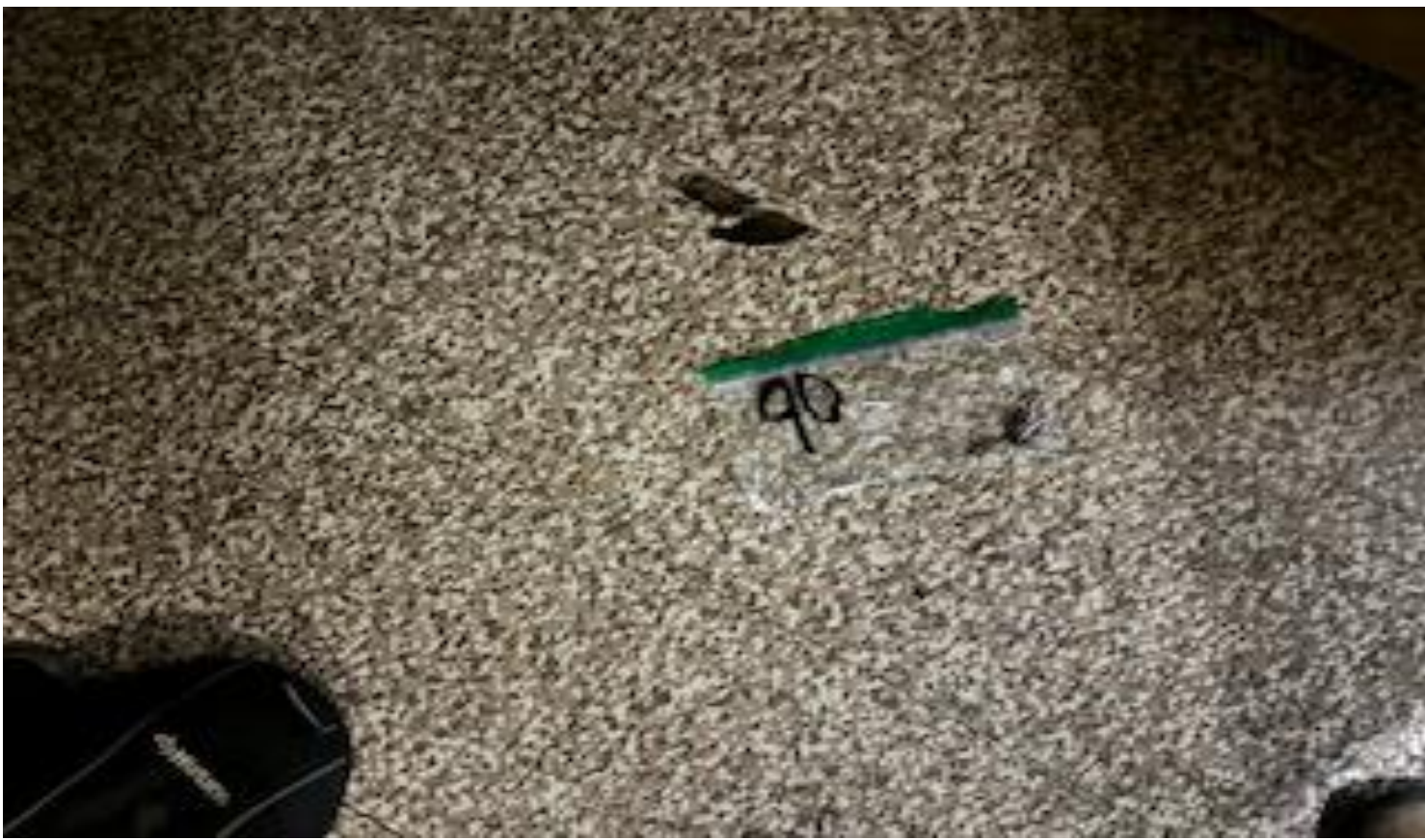
49. VIEW OF MORE REPRESENTATIVE (TYPICAL) SAMPLE OF ACM DARK BROWN 9" X 9" FLOOR TILES AND BLACK MASTIC LOCATED IN VARIOUS AREAS THROUGHOUT INTERIOR FLOORS IN BUILDINGS AT THOMAS C. MARSH PREPARATORY ACADEMY
