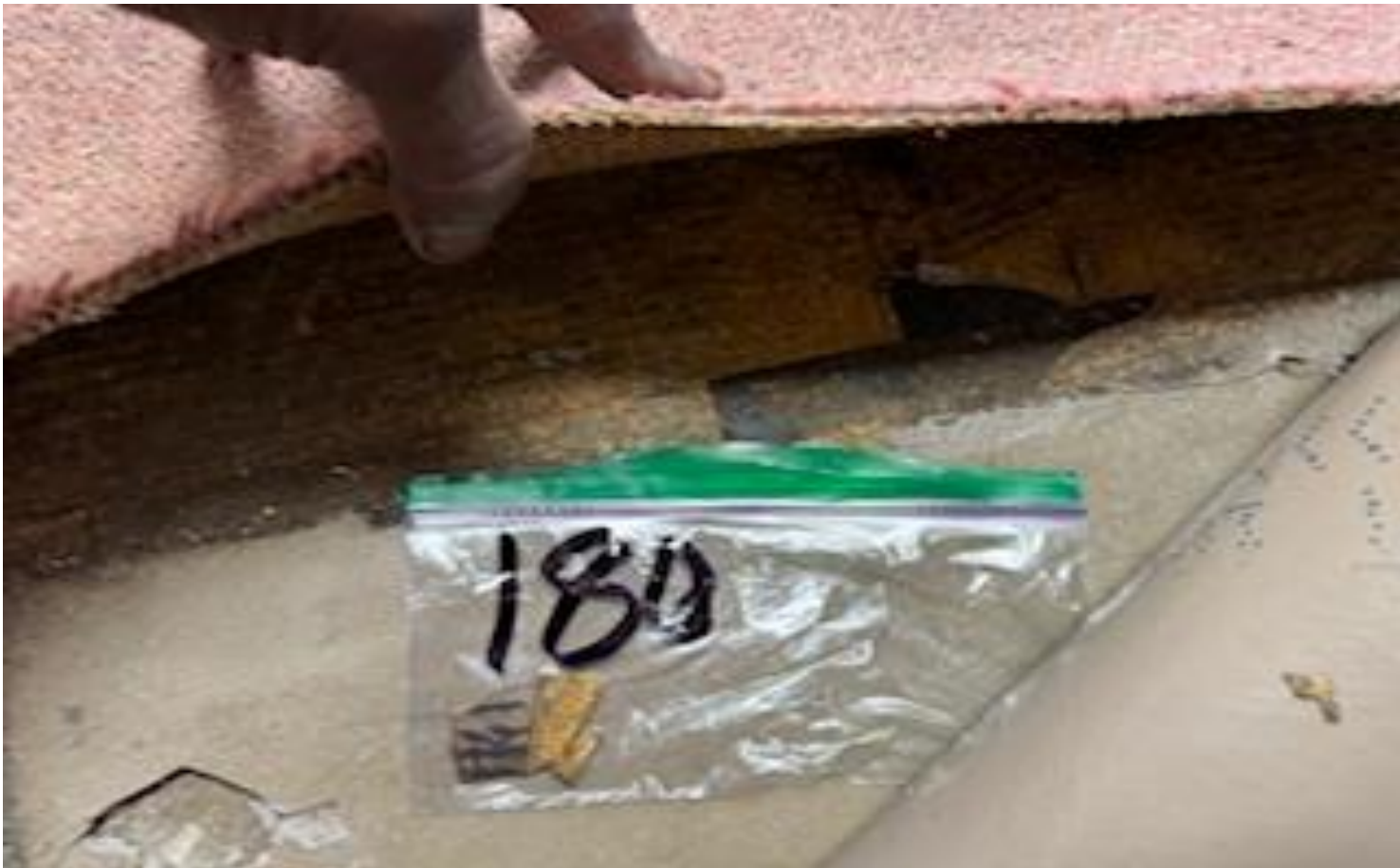
72 VIEW OF MORE REPRESENTATIVE (TYPICAL) SAMPLE OF ACM UNDER-LAYER 9" X 9" FLOOR TILES AND BLACK MASTIC LOCATED CLASS ROOMS ON THE 3 RD FLOOR SURFACES IN BUILDINGS AT THOMAS C. MARSH PREPARATORY ACADEMY
