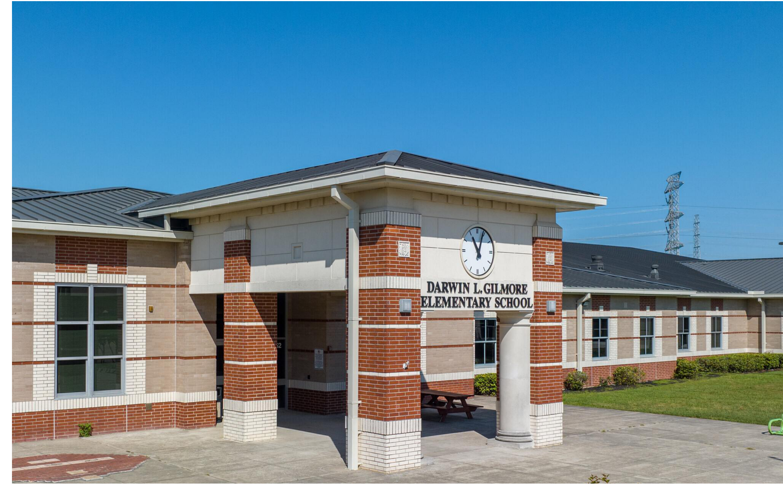
GILMORE ELEMENTARY SCHOOL
