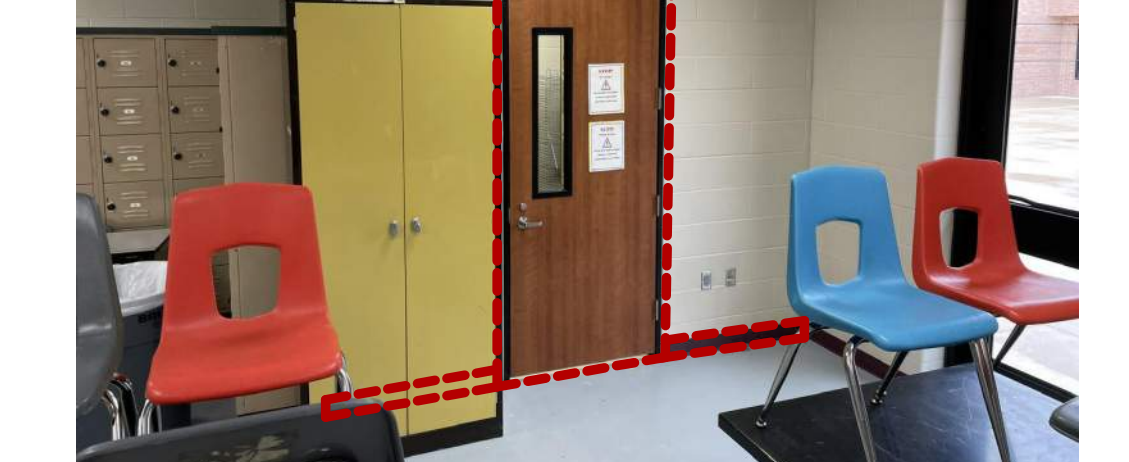
4.1 KILN ROOM WALL DEMO LOCATION
