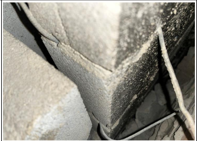
Photo 02: ACM damp proofing behind brick.
