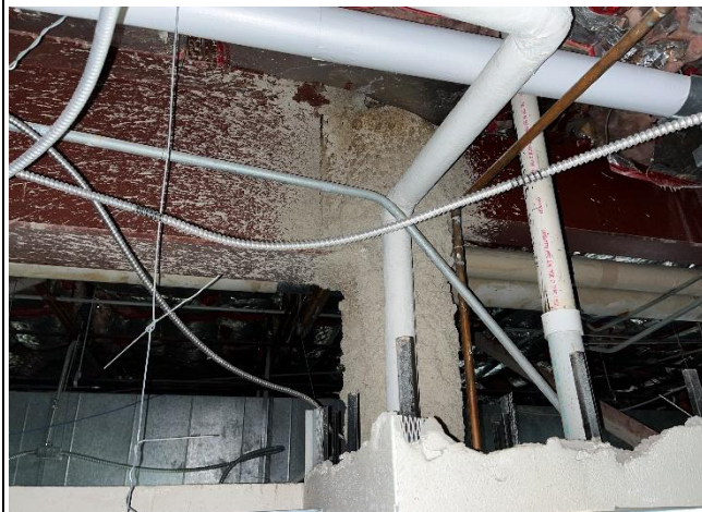
Photo 05: Fireproofing with plaster surround - nonACM
