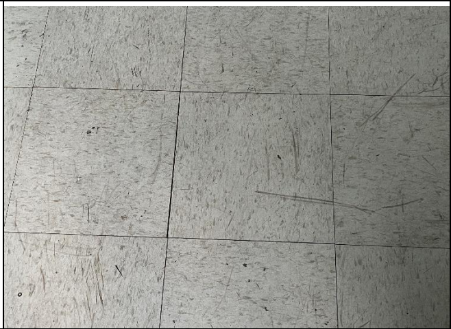
Photo 04: 12"x12" Beige vinyl floor tile with yellow mastic - nonACM
