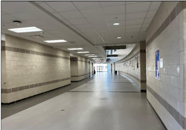
Photo 01: 16"x32" Gray vinyl floor tile with tan glue – typical - nonACM
