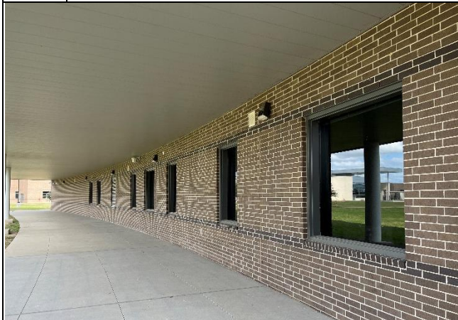
Photo 05: Damp proofing with brick and mortar - nonACM
