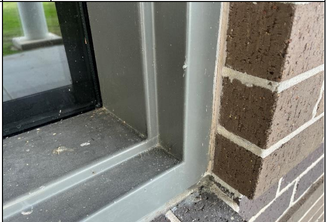
Photo 06: Window glazing putty and window frame caulking - nonACM
