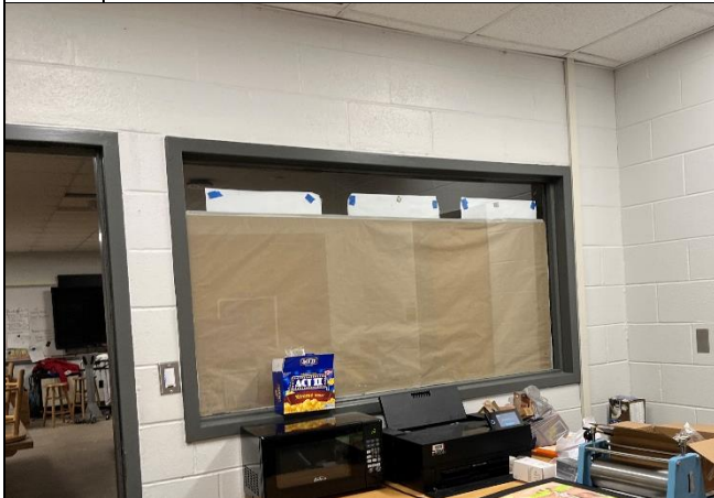
Photo 03: ACM Black Glazing Putty - Interior windows in Teacher's Office in Art Room
