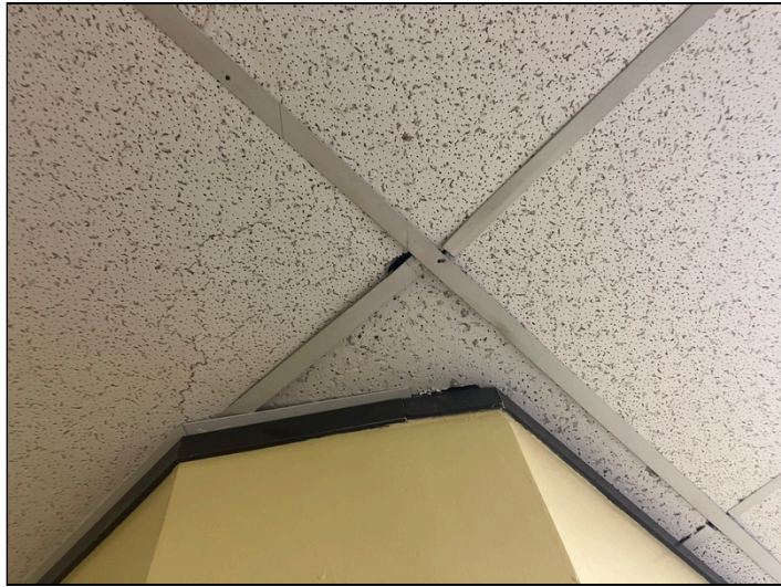
5 - Typical ceiling tile samples
