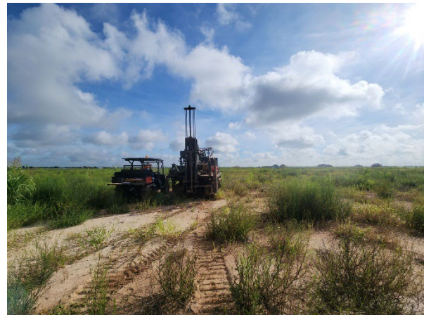
Facing North at Boring B-18
