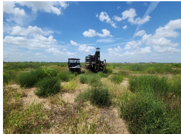
Facing North at Boring B-10
