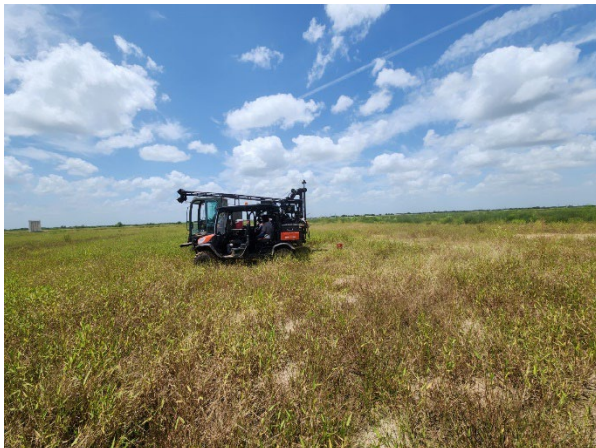
Facing North at Boring B-09
