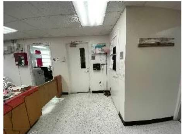
Photo #4 View of ACM vinyl floor tile (white with brown spec's) mastic (black) in the Admin Office.
