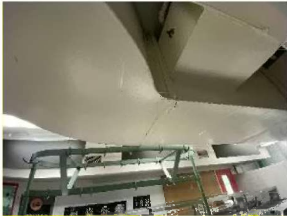
Photo #1 View of the non-asbestos containing duct mastic in kitchen.
