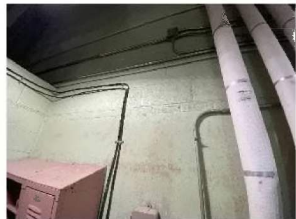
Photo #6 View of CMU block filler.
