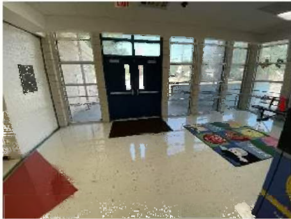
Photo #7 Interior view of the front entrance.
